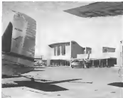
Color and panoramic cabined continuously at front door. Blue lobby, VIP suites, flight ops room, restaurants, Flight Deck Restaurant, coffee shop on second floor.
